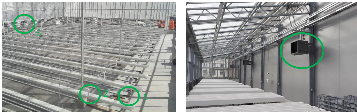
Figure 16 : Left : Greenhouse with tube of heat convector located on the soil (1) above the soil (2) and close to the wall (3) at BIGH Farm (Brussels, Be). Right: Heat convector at Gembloux Agro Bio-Tech (Gembloux, Be).
